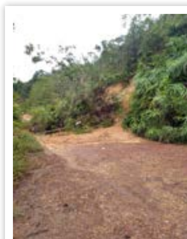
Landslide blocking roads at Hamalidah's village
