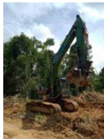
One of the many excavators used to destroy the community garden
