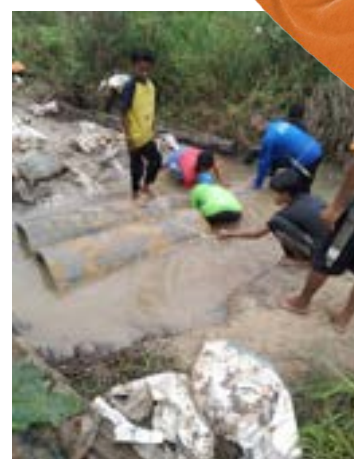
Villagers attempting to fix the damaged road with steel pipes
