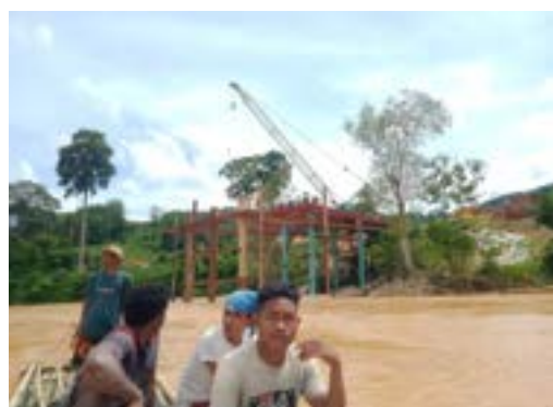
Male Temiar youths riding a raft built from bamboo while monitoring the dam construction site
